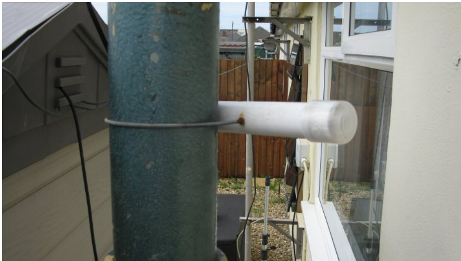
Compass is installed on the mast.
